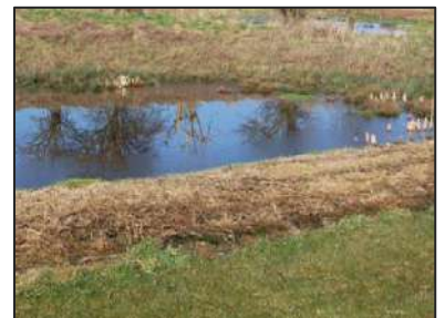
An attenuation basin, as well as allowing safe and contained storage for excess rain and storm water, could deliver opportunities for further biodiversity net gain.
